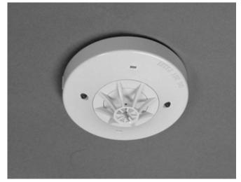
CPD-705X Ionization and Series PSD-715X Photoelectric Smoke Detectors when using multifunction base configuration.
